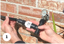
1 Connect in order: filter (A) to pressure regulator (B) to hose swivel (C); Attach unit to garden hose or faucet; Attach poly supply hose (D) to hose swivel (C)
