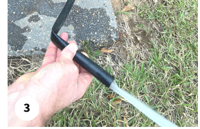
3 Flush the system before closing the ends of the poly supply hose (D).
