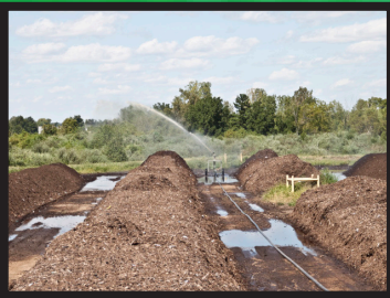
Waste Water Reuse
